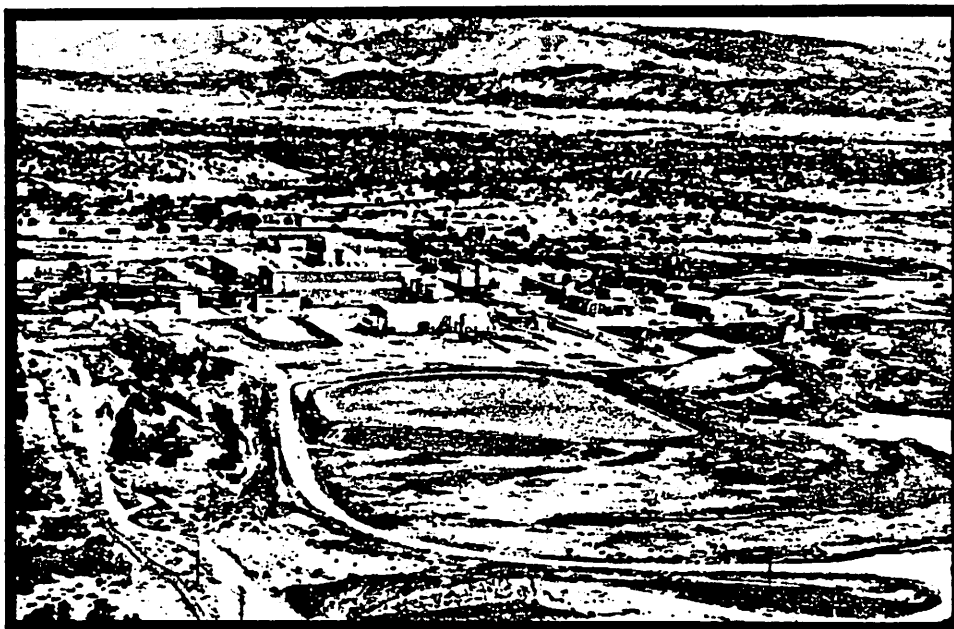
Cotter Uranium Plant with leaking tailing ponds.
